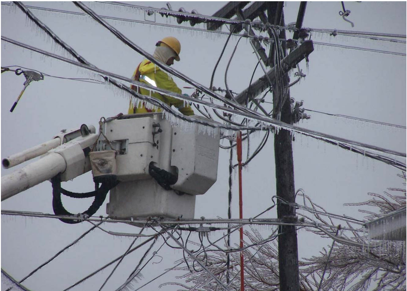
A worker repairs a powerline following a 2010 ice storm in Joplin.
